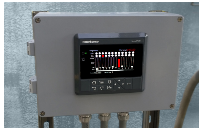
B-PAC ultra-rugged (field-mountable) user interface displays diagnostics (data also available over Fieldbus).
